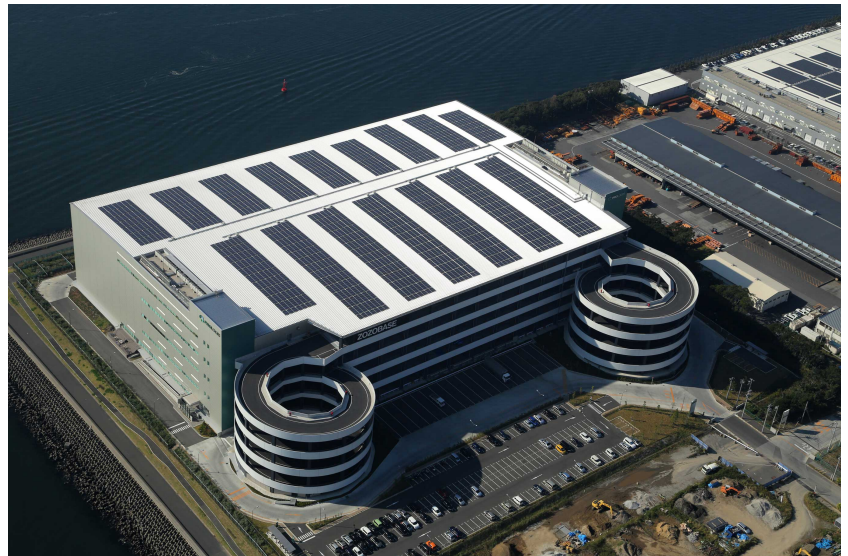
Prologis’s Multi-Story Warehouse in Narashino, Japan. Source: Prologis, Inc. www.prologis.com
